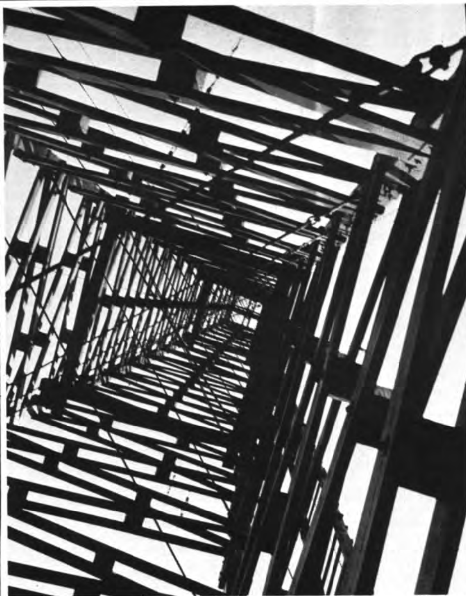
The "Great Storm" of Nov. 25th 1901 blew down the original circular masts, one nearly hitting Mr. Vyvyan, Marconi's Assistant. The Second towers erected consisted of 4 units built on a square each 200 feet apart. They were built of 3x12 timbers bolted together and set in a concrete base 30' square by 4' thick. The masts were 210' high, starting at 24' square at base and tapering to 8' at top. When built the Easternmost tower was 165 from the edge of a cliff overlooking the Atlantic. By 1906 it became evident erosion of the bank would destroy them but by then the station had already become obsolete.
